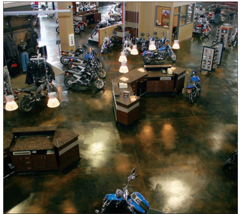
This Harley Davidson store in St. Charles, Illinois, had its floor chemically stained with black, reddish brown, and light green colors in a random, free-style fashion.
