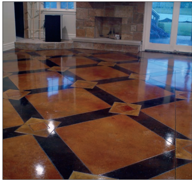
This residential floor has been chemically stained with dark brown, amber, and yellowish green colors. The pattern was cut using a 102-mm (4-in.) diamond blade on an angle grinder, typically 3.2 mm (0.125 in.) deep. Saw cuts prevent the different colors from bleeding together.
