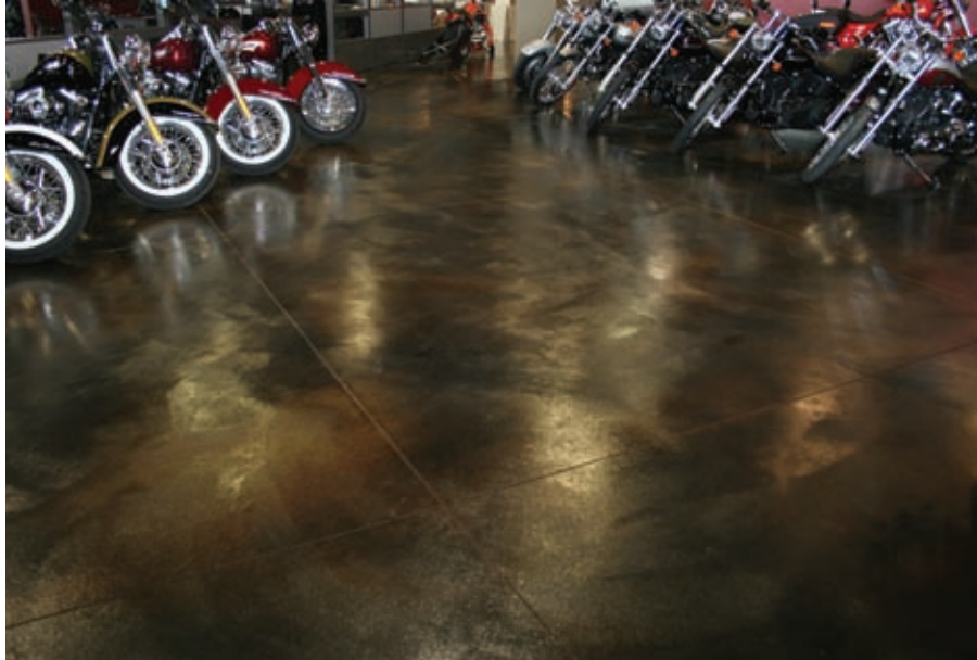
Chemically reactive stains and, to a lesser extent, non-reactive stains or dyes will produce color variations. The degree of variation is a function of concrete porosity, texture, age, application method, and the original color of the substrate.
