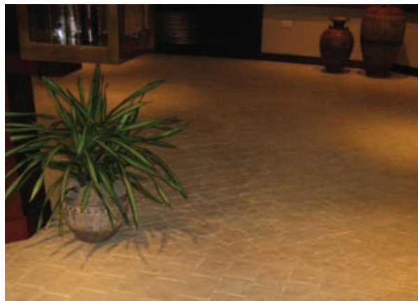
Application of a protective sealer is usually recommended for stained surfaces. Periodic application of a maintenance wax, in turn, protects the sealed surface from scratching, excessive wear, or damage.
