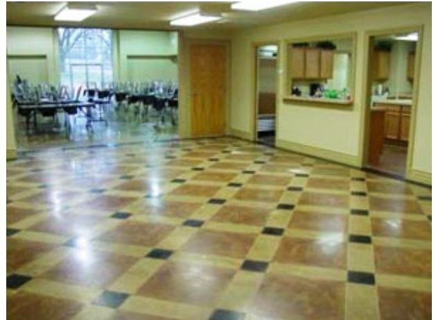
Polished concrete, combined with patterns and stains, provides attractive, durable and environment friendly floors (Photo Courtesy of Concrete Décor)
