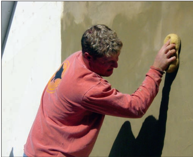
In the above photos, this application is using a damp sponge to gently rub the scratch coat's surface before it completely dries. The result is a 'sanded' finish that matches the weathered appearance of actual brick mortar.
