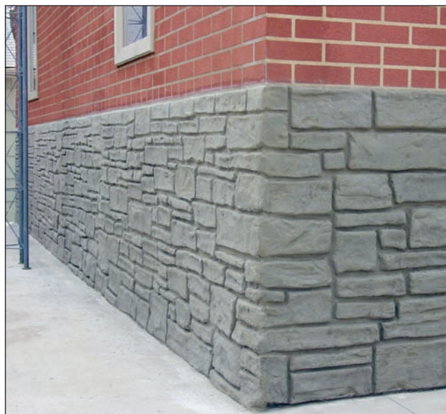
The carriage house's finished wall is evocative of the budding Ottumwa community in 1865.
