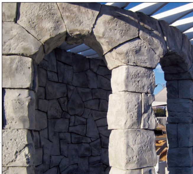
The technique of hand-carving can be used to create a more custom 'stone' effect, as shown in the above photos.
