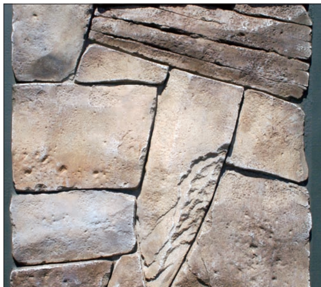
The technique of hand-carving can be used to create a more custom 'stone' effect, as shown in the above photos.
