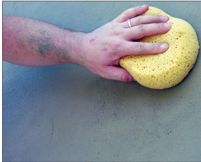
In the above photos, this application is using a damp sponge to gently rub the scratch coat's surface before it completely dries. The result is a 'sanded' finish that matches the weathered appearance of actual brick mortar.
