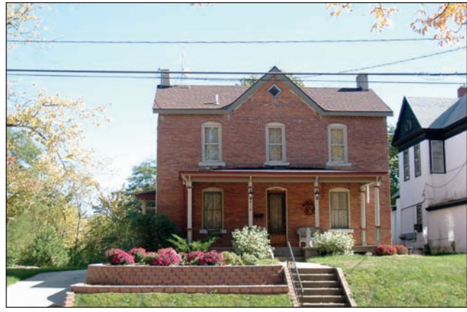
Before and after: Prior to sand-blasting, the Thomas Healy House was painted white (left). Sand-blasting gently removed the layers of paint from the brick and stone to reveal the house's rosy brick and natural limestone (right).
