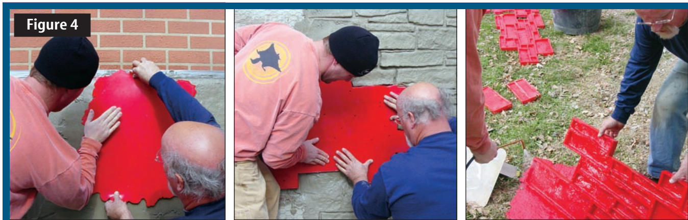
Figure 4 The surface is first textured (left) and then imprinted with a stamping tool (center). A liquid release agent is spray-applied to the wall mix and tools prior to use (right). Depending on humidity, temperature, and overlay, stamping can take up to an hour.
