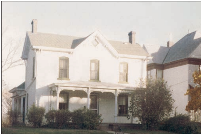
Before and after: Prior to sand-blasting, the Thomas Healy House was painted white (left). Sand-blasting gently removed the layers of paint from the brick and stone to reveal the house's rosy brick and natural limestone (right).
