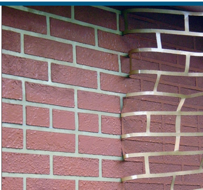
The topcoat is gunned over the stencil and scratch coat (left). Once the topcoat dries, the stencil is pulled away (right).
